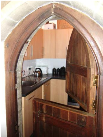
2009 Funding for major project. Vestry extension, toilet facilities, kitchenette, levelling of floor and carpeting across Transepts and crossing. Friends' contribution: £13,000
