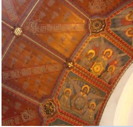
1999 Redecorate Chancel, clean stonework and ceiling paintings and install uplighters £6,246
