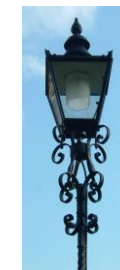
2004 & 2015 Restoration and relocation of churchyard lampstand, plus repair to base. Installation of time clock for this and porch light £3,179
